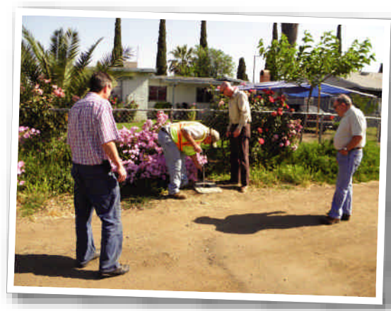
Construction (top) and final inspection (above) on the Fairways Tract connections.
