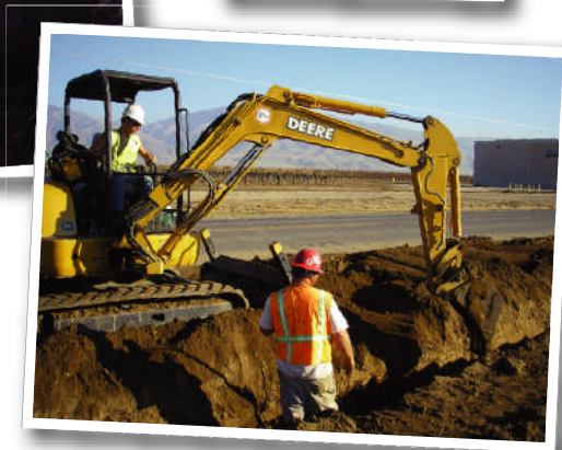
12 inch main water transmission pipeline was installed to connect the Edmundson Acres community to the Arvin CSD water system.
