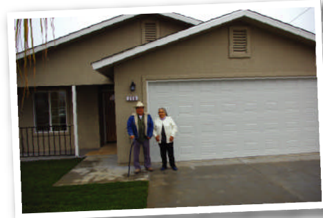
A 91 year-old home gets a new beginning for its 81 year-old owner! (Rehabilitation)
