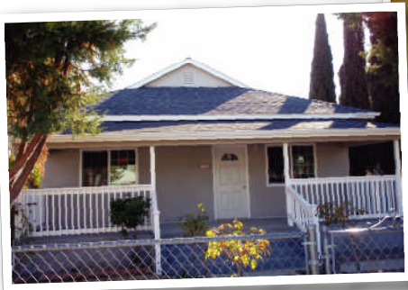
A brand new safe home! (Reconstruction)
