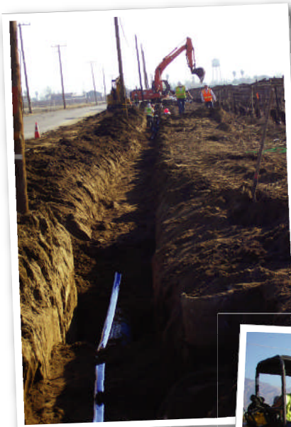
12 inch main water transmission pipeline was installed to connect the Edmundson Acres community to the Arvin CSD water system.
