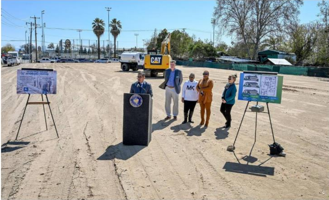
Fresno Councilmember Miguel Arias, at lectern, is joined by representatives from Self-Help Enterprises, the Fresno Redevelopment Successor Agency, and the Golden West Side Planning Committee, announces the beginning of construction of a single-family affordable housing project on an empty lot near Edison High School at Walnut and Florence avenues in west Fresno on April 4, 2023. CRAIG KOHLRUSS ckohlruss@fresnobee.com
