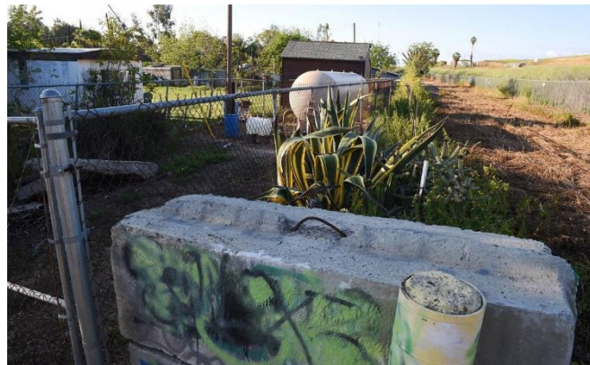
One of two water wells, background, is located behind fencing between a private home at the end of Morgan Road, a gravel road one block long, and a canal delivering water south.
