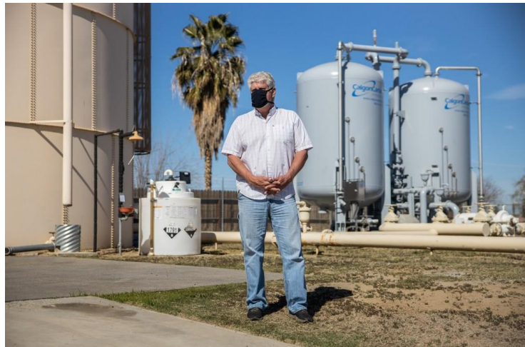
Scott Taylor, General Manager of the Lamont Public Utility District at Well #13 in Lamont, which recently broke down after installation of a $1 million treatment system for 123-TCP.
