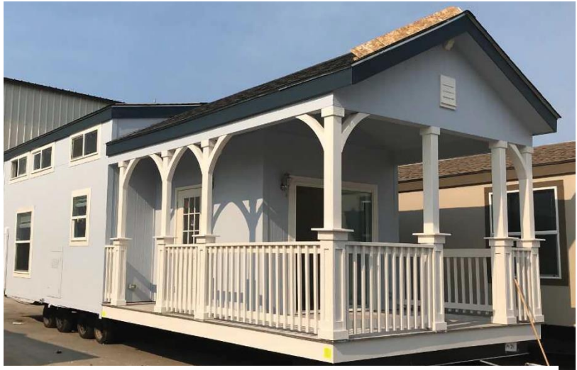
Each of 52 pre-fabricated homes will include a bedroom, restroom, kitchen and laundry room.
