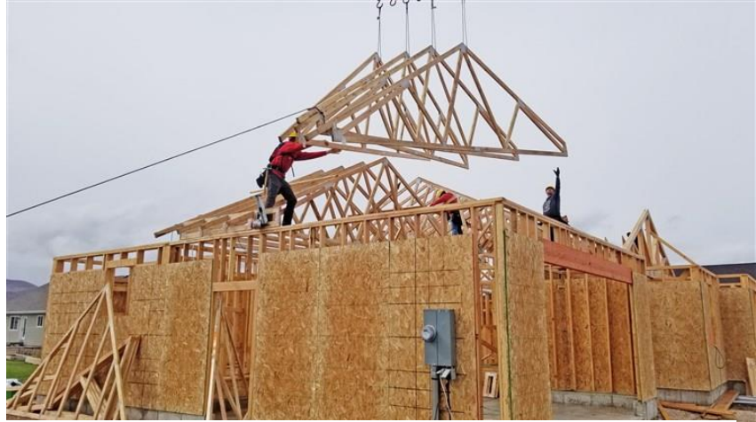
Members of Self-Help Homes build a home in Heber City, Utah.
