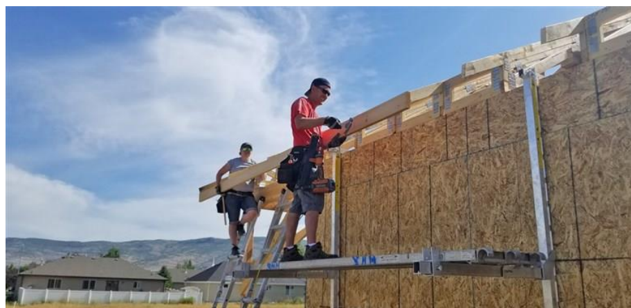
Lisa and Craig Godfrey construct their house in Heber City, Utah.
