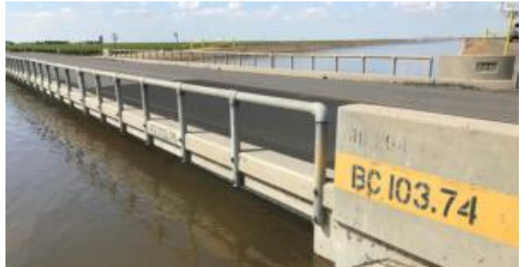
Prop. 3 will provide $750 million to fix subsidence issues caused by overpumping during the drought. Near the Tulare County, Kern County border, bridges crossing the Friant-Kern Canal have sunk 3 feet in as many years.
