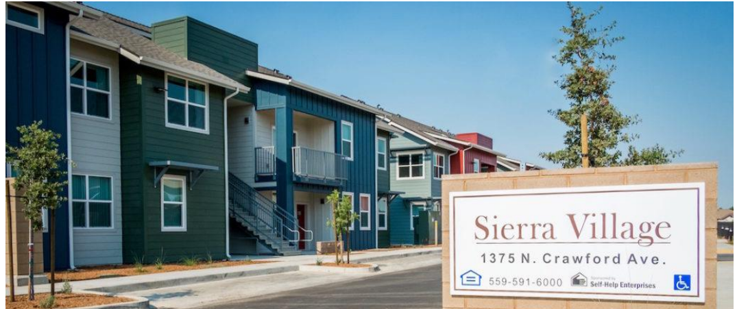
Sierra Village, at 1375 N. Crawford Ave. in Dinuba is a highly energy efficient and transit-friendly project built by Self-Help Enterprises.
