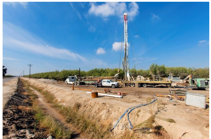
A water well being drilled in an almond orchard in California's San Joaquin Valley. Drought has increased groundwater pumping, causing shallower wells to run dry. (Citizens of the Planet/Education Images/UIG via Getty Images)
