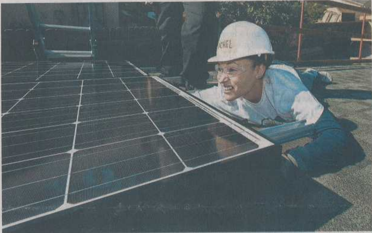
Rachel Murillo connects power leads as other volunteers add solar panels to a Self-Help Enterprise project in Tulare. RON HOLMAN
