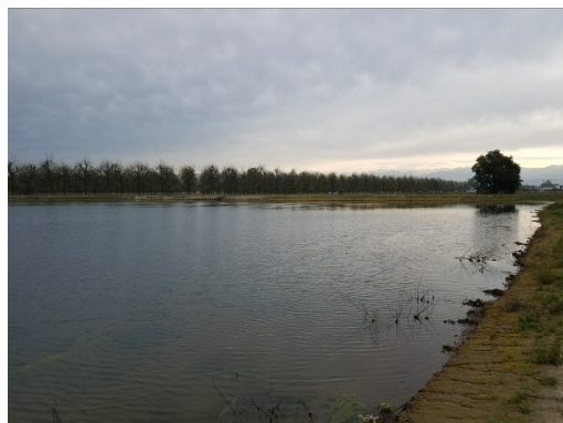
Groundwater Recharge Basin
