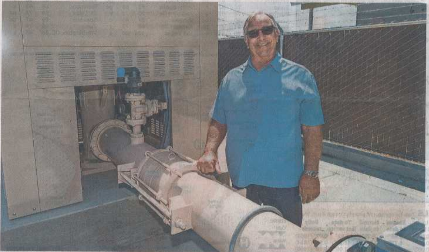
Tim Doyle stands with the nearly operational pump #45 on South I Street in Tulare on Tuesday. It is expected to provide 1,100 to 1,200 gallons per minute. PHOTOS BY RON HOLMAN
