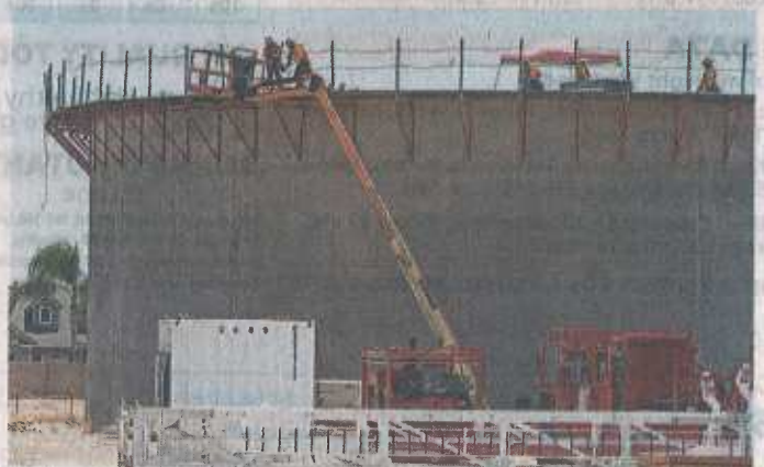
A 2-million-gallon water tank is under construction on Alpine Avenue in Tulare on Tuesday.
