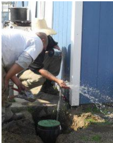
Workmen hook up the last home in Phase 2 of the East Porterville Water Supply Project in early February. The total number of homes hooked into the system through phases 1 and 2 total more than 750. Courtesy/Self-Help Enterprises
