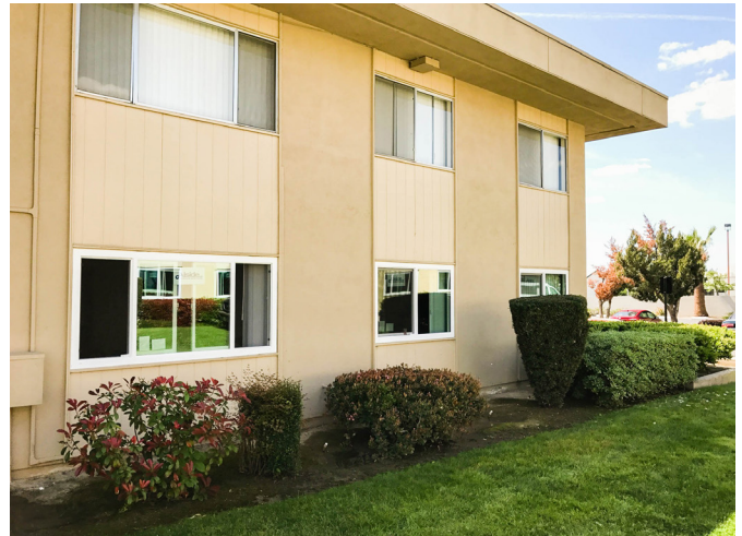
Old windows (top) all being replaced with new dual-pane, energy efficient windows (bottom) at the North Park Apartments in Oildale, CA.
