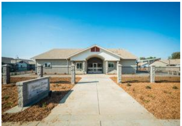
The Highland Gardens Community Center (Photo Credit: Self-Help Enterprises)
