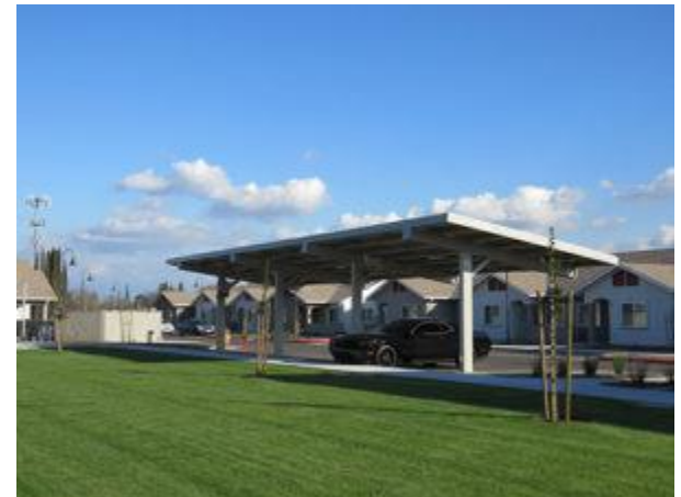
Solar Carports located next to green space at Highland Gardens. These carports provide shaded parking for residents and generate renewable energy to lower utility costs. (Photo Credit: Self-Help Enterprises)
