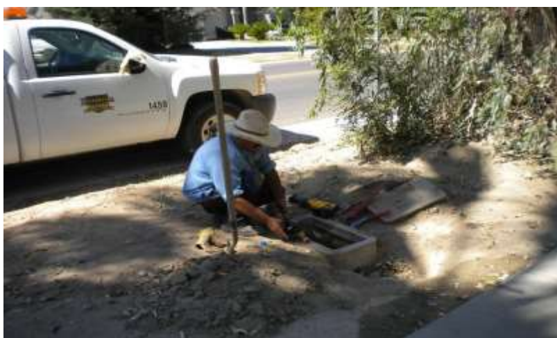
City employee Manuel Ramirez installs a water meter in Kerman.
