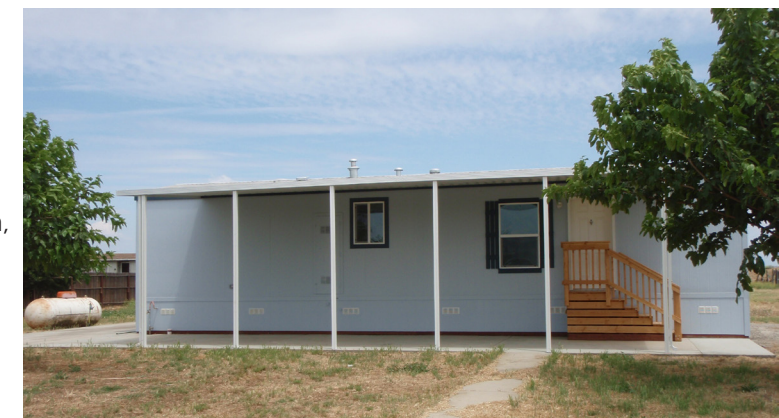
Top. Ms. Stark's unsafe home. Bottom. Ms. Stark's new, safe manufactured home.
