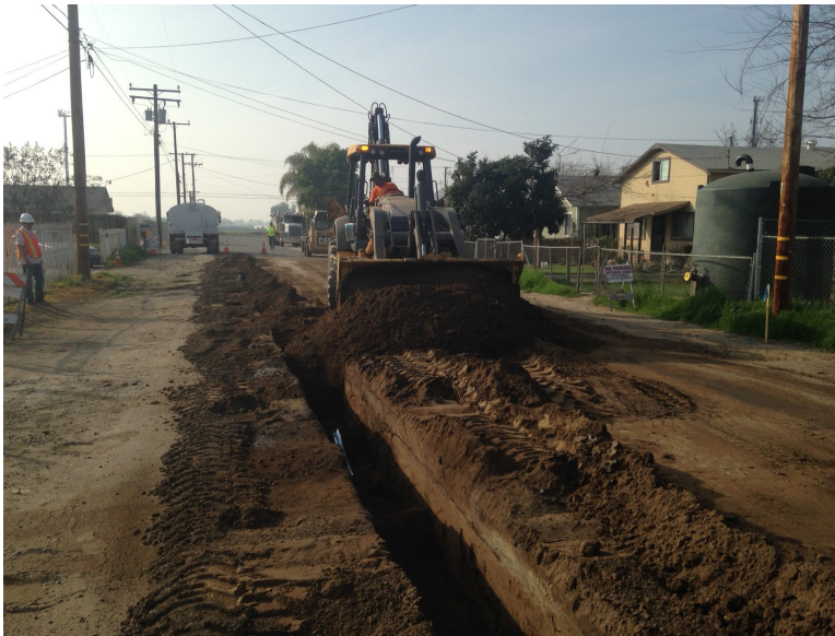
Bottom. Cameron Creek: Construction of a water line in Cameron Creek Colony that connected nearly 100 homes to the City of Farmersville water system.
