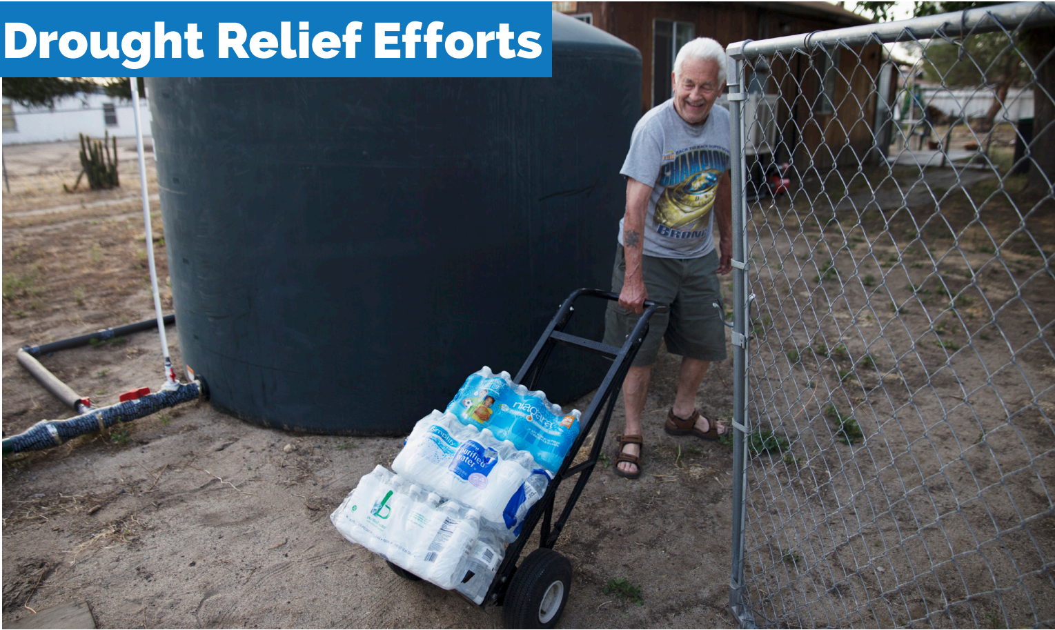
Top. Emergency Water Tank: The pressurized water tank system provides water to the Chavez home in East Porterville.
