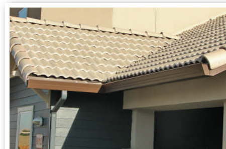
Cool tile roof reduces energy demands
